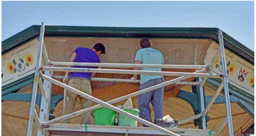
Pictured from left to right are; Alex MacKenzie and Matt Cook applying the scraffito to the Clevedon bandstand.
