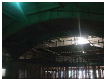
Work in progress King Edwards's Hotel
